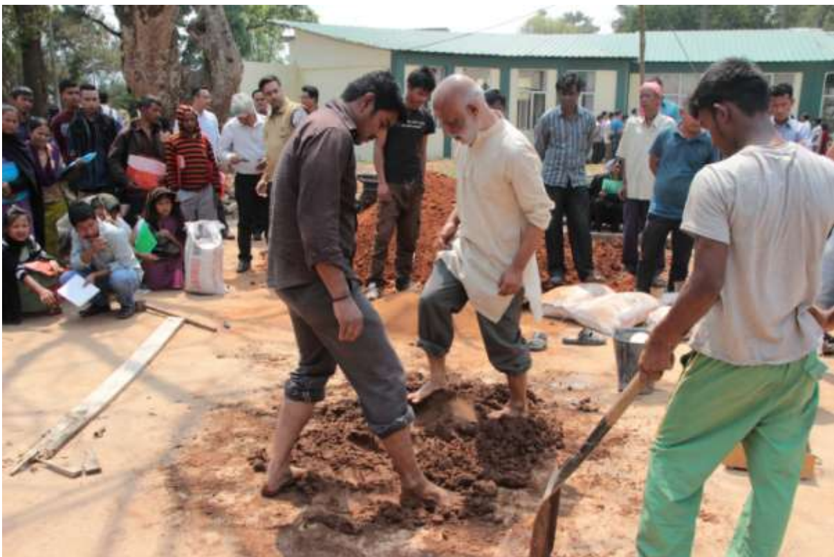
Picture 9 Pugging of the soil mix which will be used to make the stabilised adobe blocks. Demonstrated by the team from Gramavidya.
