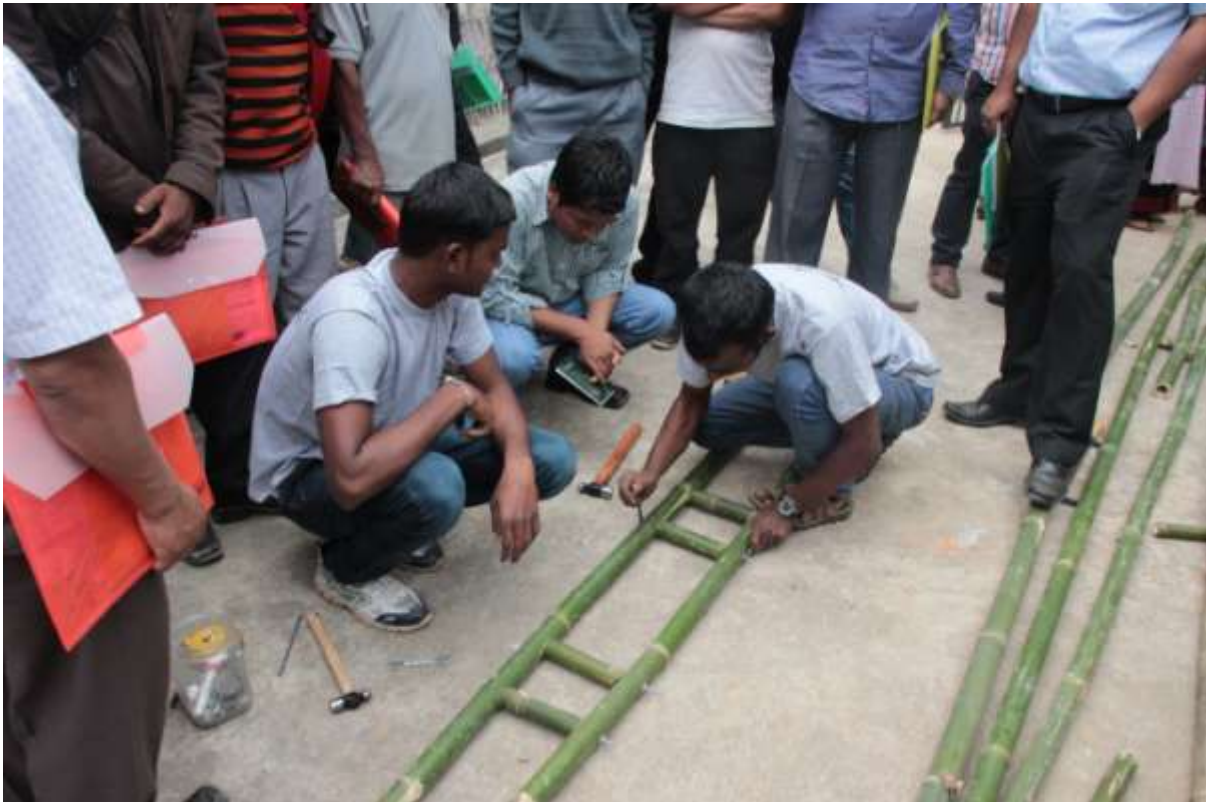
Picture 21 Assembling a bamboo member that can be used for as a column or as a beam.
