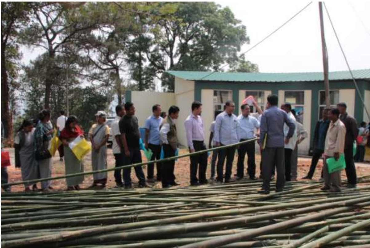
Picture 17 Selecting the appropriate bamboo for construction.
