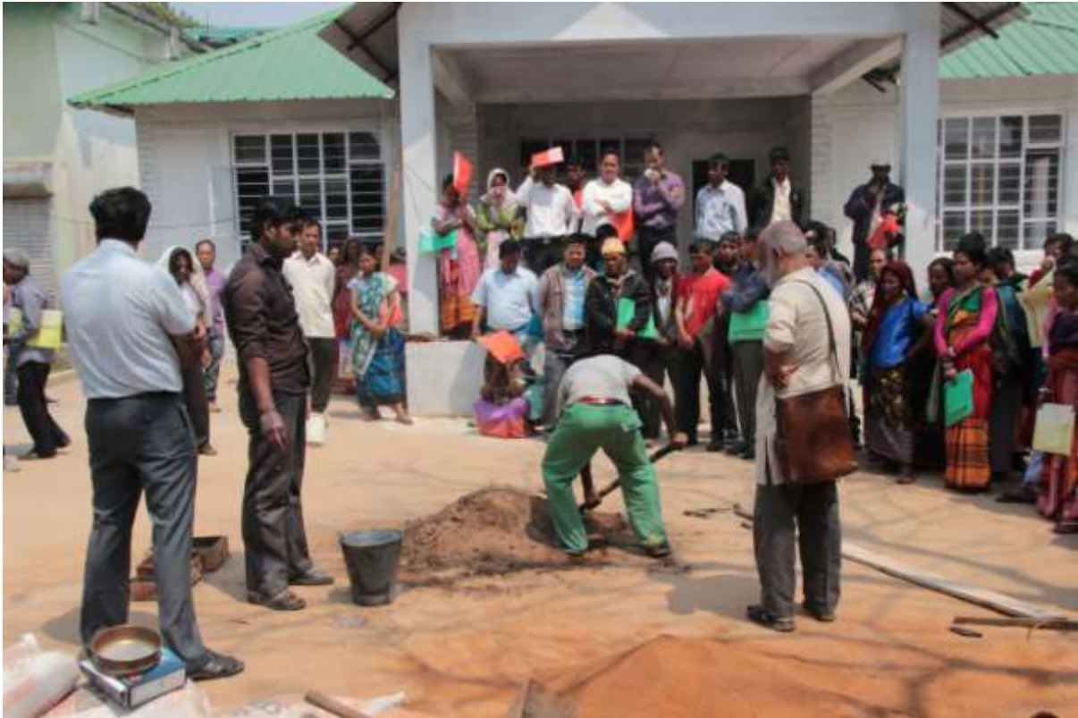
Picture 8. Mixing of the soil cement mix using the lime water.
