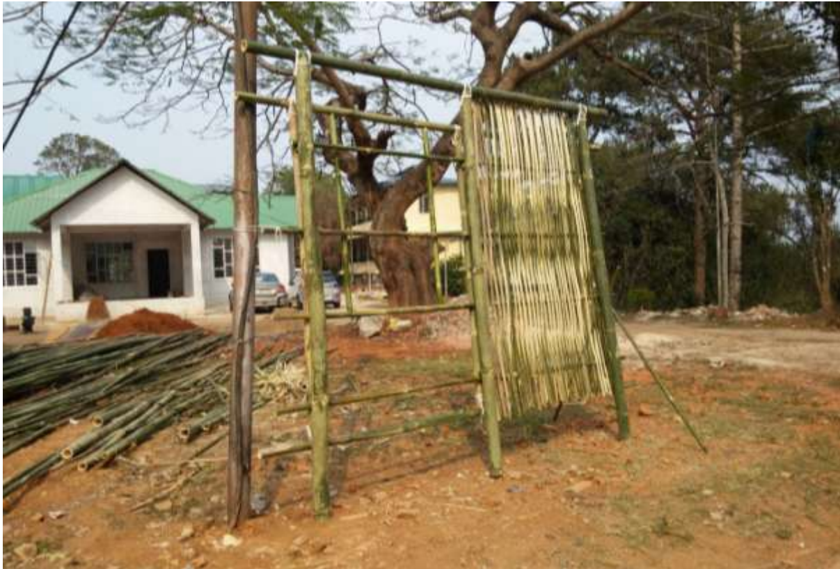
Picture 25 Bamboo walling panels assembled using large dia. Members for the main vertical and horizontal members and smaller dia. Members for the walling panel secondary members and split bamboo used for the walling weave.
