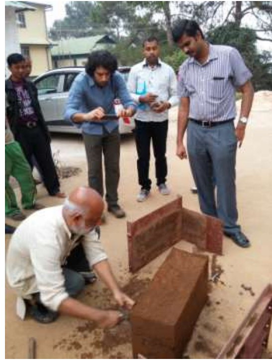
Picture 15 Rammed Earth Production being demonstrated.
