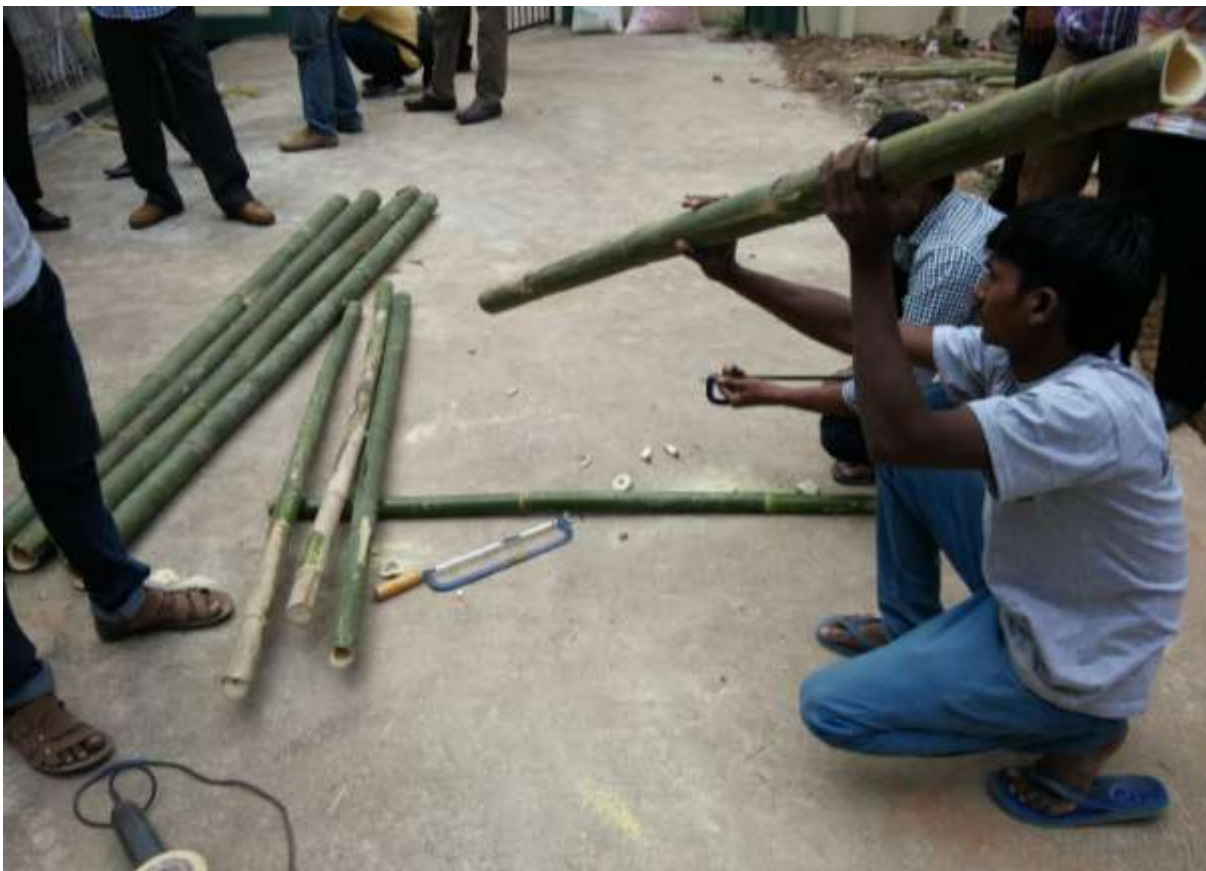
Picture 19 The sorted bamboos being sized for fabrication
