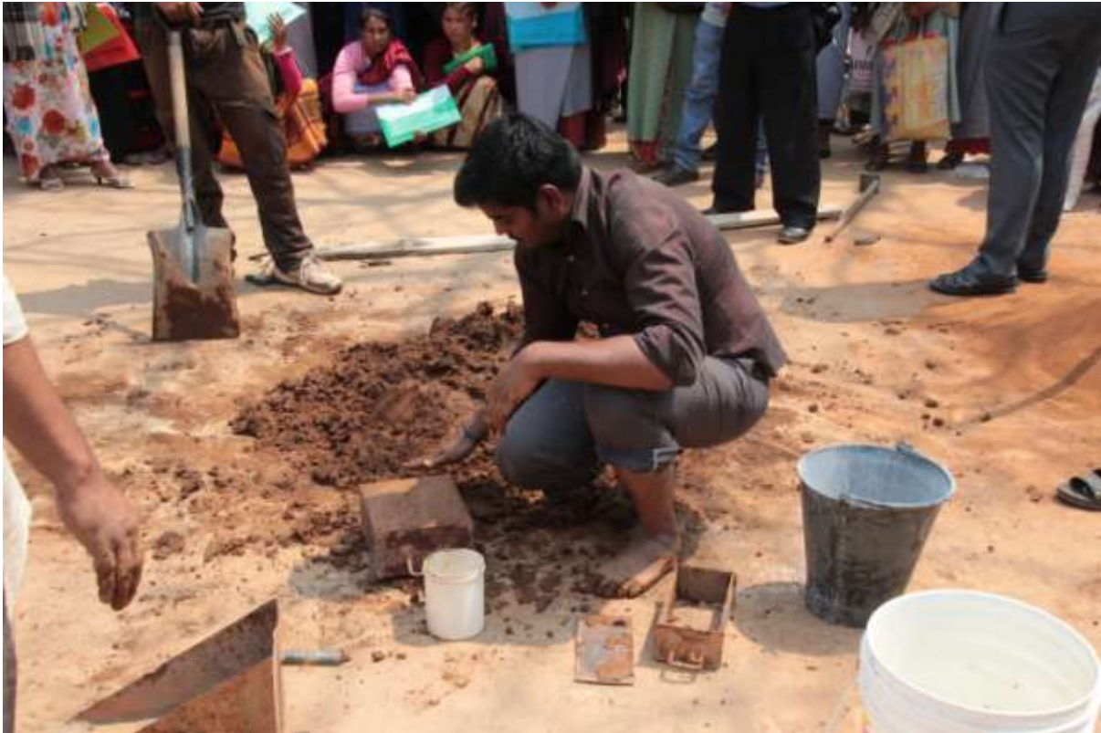
Picture 10 Filling the mix into the mould
